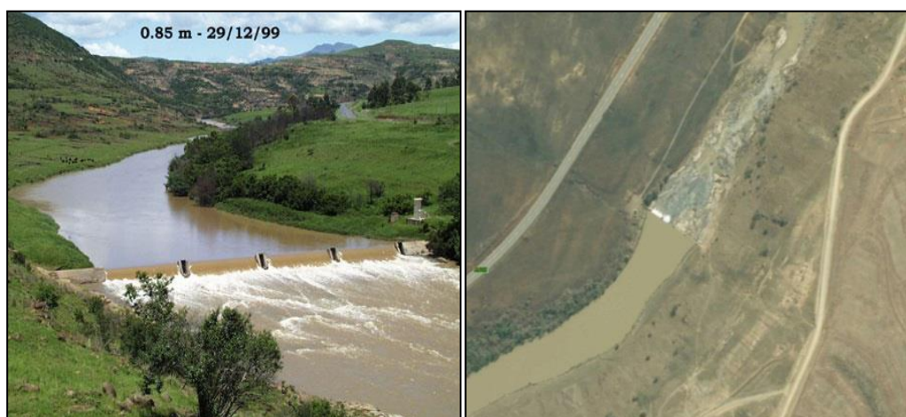
Figure 3.1: Flow gauging weir U1H005
