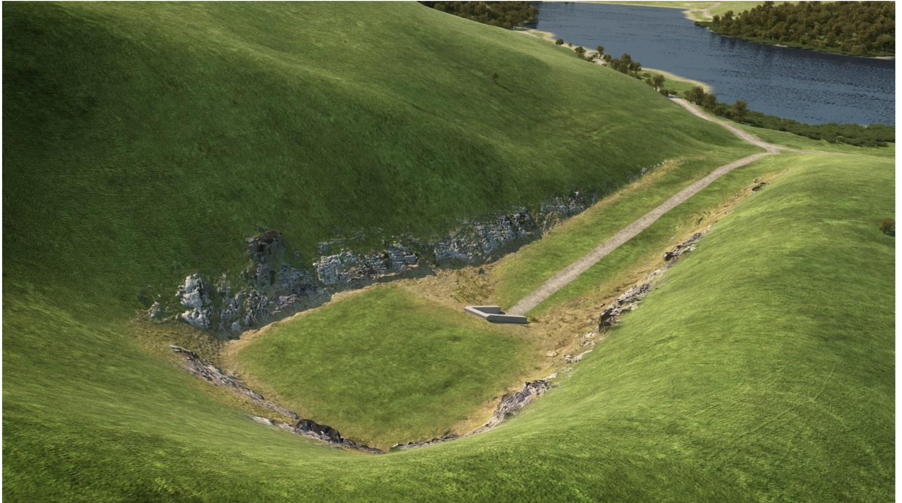
Figure 4.17: Three dimensional artistic impression of the tunnel outlet in the Baynesfield valley - View 3
